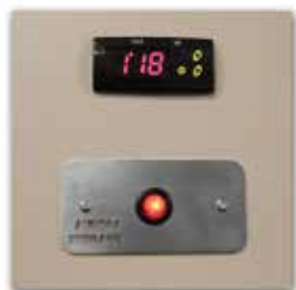
Separate thermostat and fan control on door.
